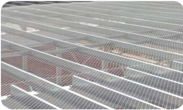
The SKY-WEB® II system offers complete passive protection at the leading edge of roof to workers installing roof systems.
