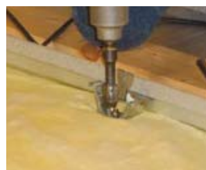
BUTLER® Pre-punched purlins offers precise installation
