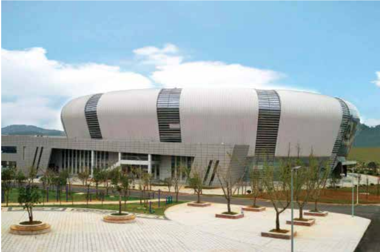
Stadium with Lysaght Flexlok - Concealed Fixed Roofing System
