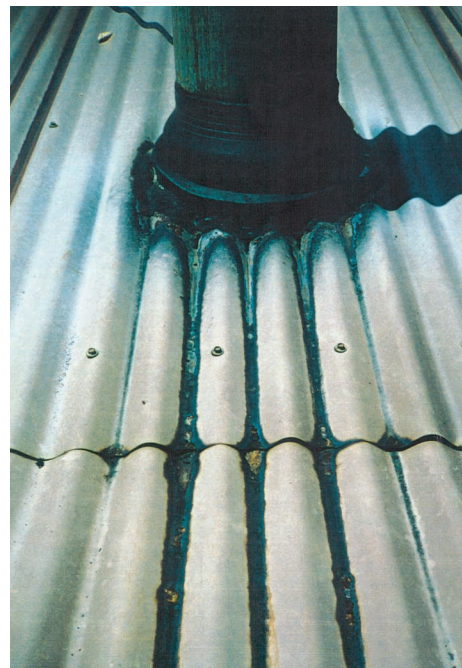
Figure 1: Flue Deposition/Corrosion.
