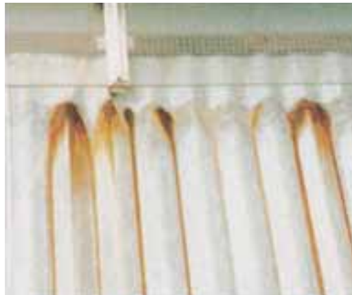
Zinc-coated roof receiving water from glass roof.
