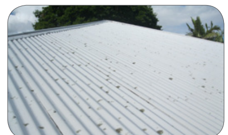
Figure 4: Photograph of a roof made from COLORBOND® steel showing spotty lichen and fungus growth spread across the structure.
