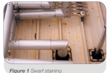
Figure 1 Swarf staining
