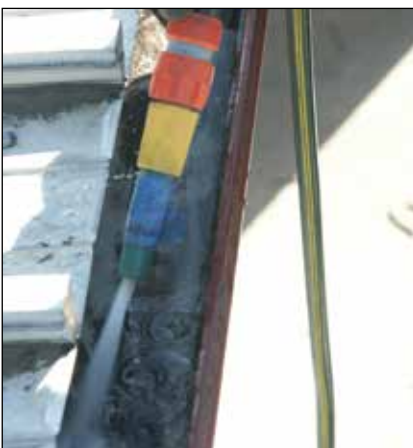
4) Spray the gutter & downpipes with water to soften and break up the dirt.
