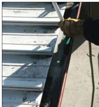
5) Use a soft bristle brush and sweep the dirt out. Rinse again.
