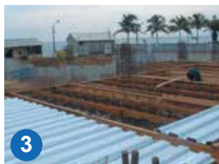
3 Place on steel or concrete beam
