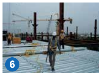
6 Fix SMARTDEK® 51 profiles to steel or concrete beam
