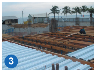
3 Place on steel or concrete beam
