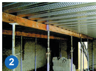
2 Place temporary support if required
