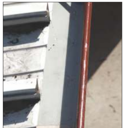
6) When the gutter has been cleaned, it should look like this.
