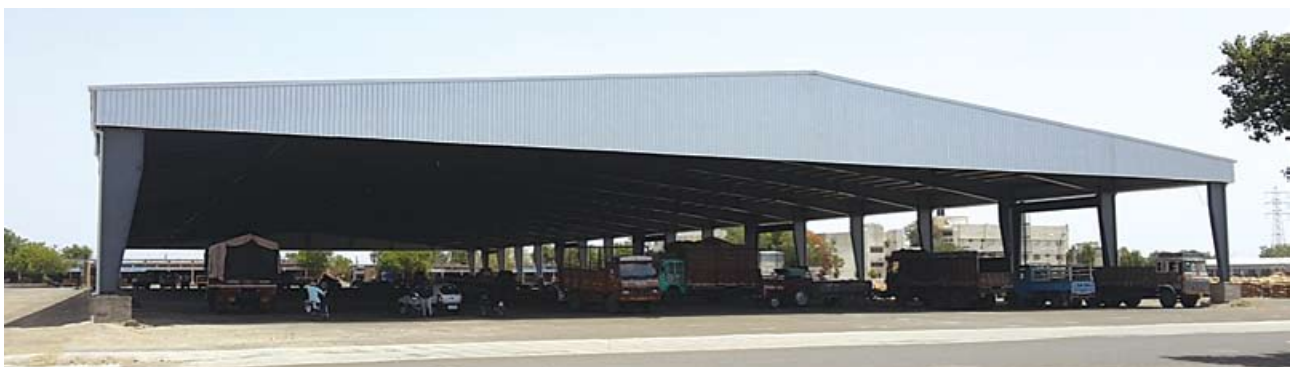
200 feet clear span
