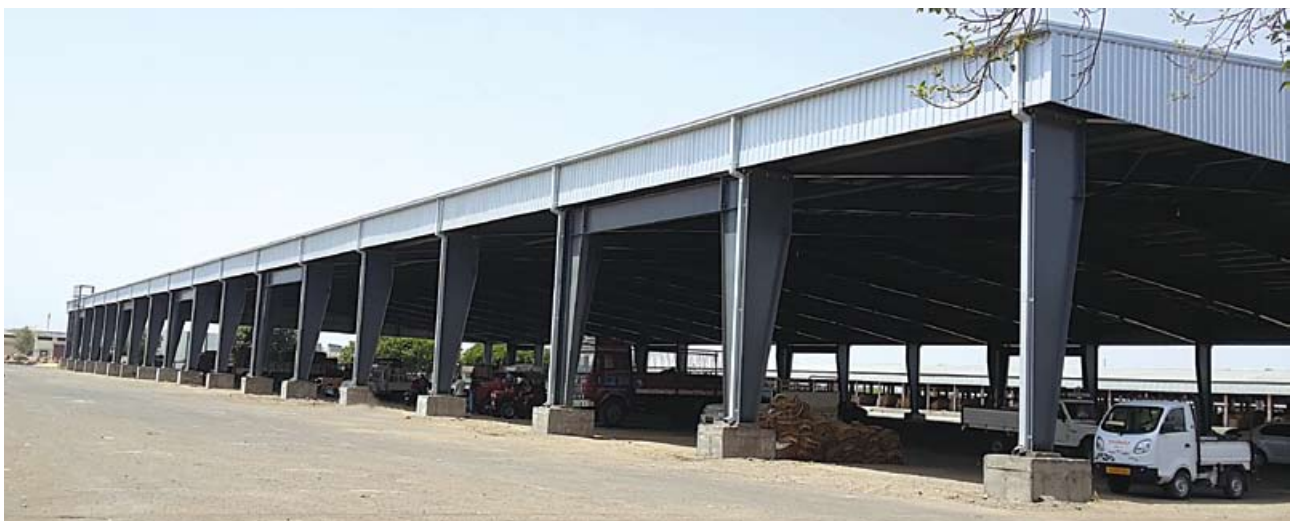
500 feet long building with 29'6" Bay spacing
