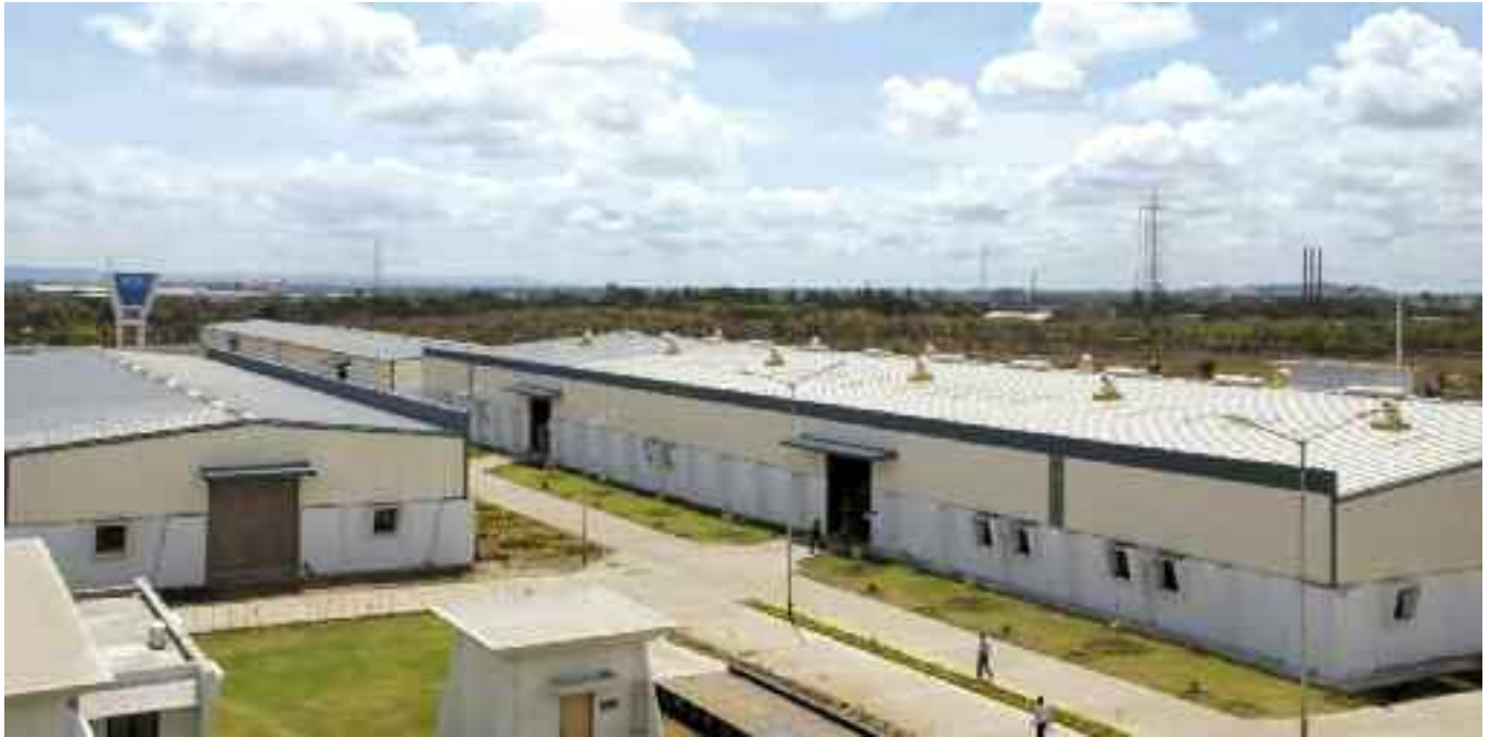
Five BUTLER® Buildings were supplied to Arc Tec Systems Limited
