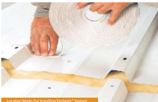
Location Marks For Installing Panlastic® Sealant
