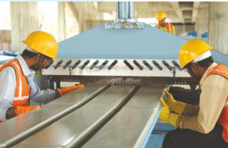
On-site crimping, an Innovative approach to achieve operational and product excellence with cost optimisation
