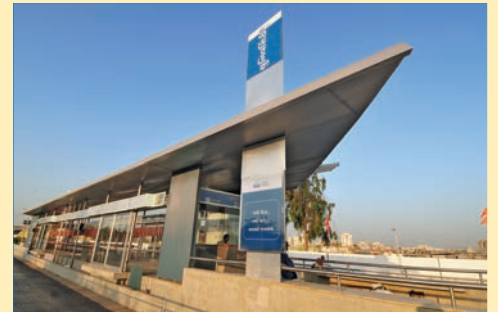
Bus Stop False Ceiling
