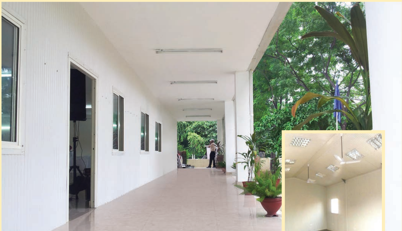
Corridor Wall Panel
