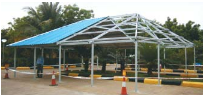
Test site, Tata BlueScope Plant, Sriperumbudur (Tamil Nadu)
