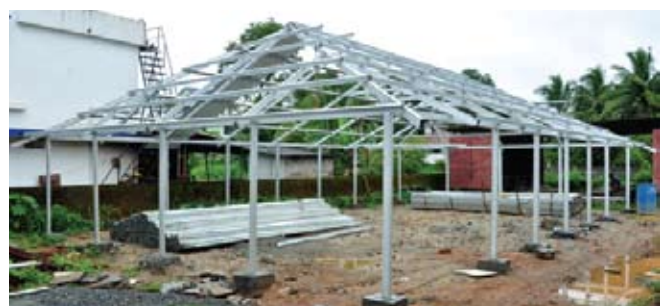
Stock Yard (Under Construction), Palakkad (Kerala)
