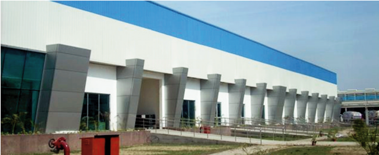
Hindustan Unilever Limited's Mega Project Delivered in 60 Days
