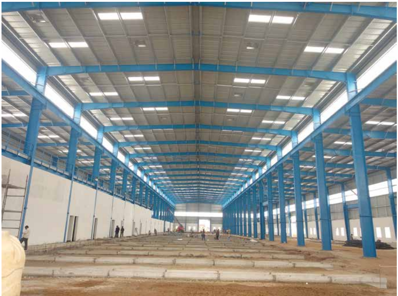
Safe erection practices at Hitech Corporation facility in Mysore
