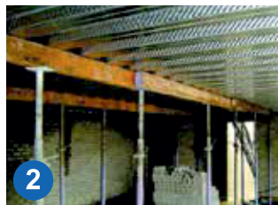
2 Place temporary support if required
