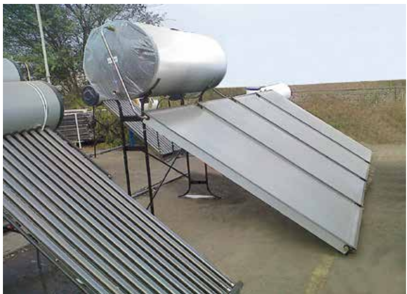
Solar Water Heaters
